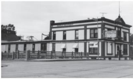
↑ Pictured above is a 1969 photo of the Western Products building.
